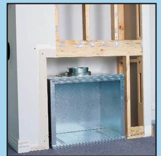
Zero Clearance Box positioned in framework on 12mm sheet
