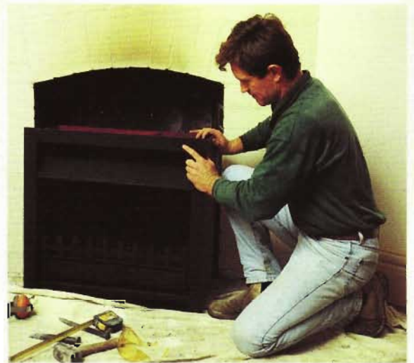
2. Choose the appropriate firebox from a range of sizes
